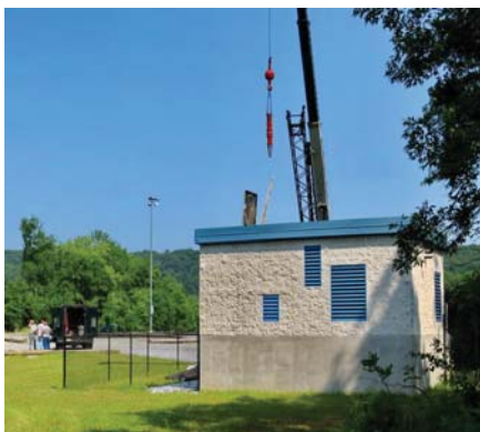
New Well House - Well Pump Installation (2014)
